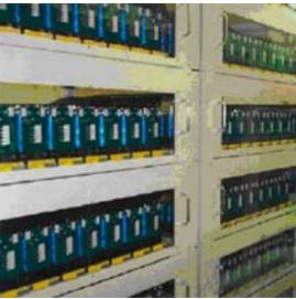
Fig. 23. Large electrochemical capacitor storage system that provides short-time uninterruptible power. (Photo courtesy of Nippon Chemi-Con)
