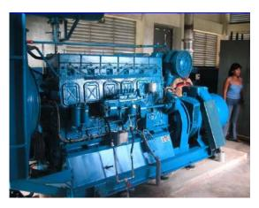
Fig. 6. 100-kW diesel generator.
